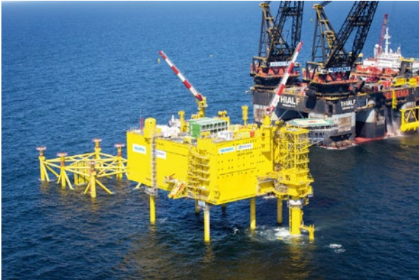
Figure 4: The HelWin2 project includes the realisation of a 690 MW grid connection for wind farms near Helgoland
